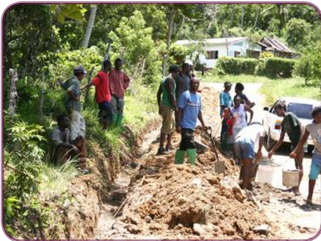
Community labourers working on their project
