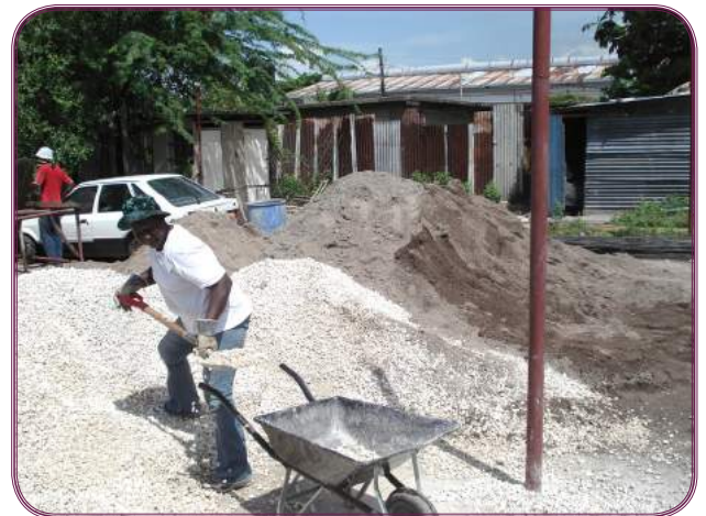
Resident of Whitfield Town working on the Zinc Fence Removal project.
