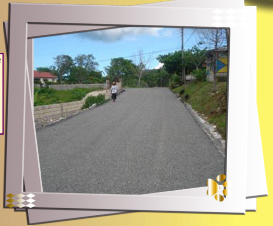
Commodore Road in Portland before (left) and after (right). One of 15 agricultural feeder roads that were damaged by hurricane Dean and rehabilitated by JSIF
