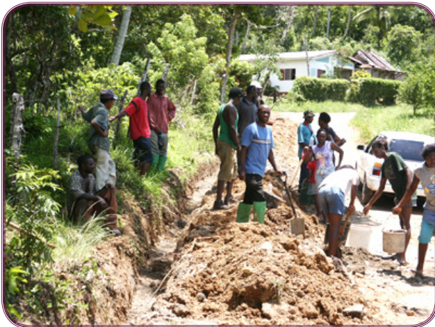
Community labourers working on their project
