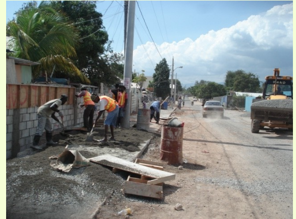
Zinc fence removal in progress at Federal Gardens
