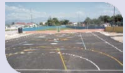
The completed court at the Portmore Park - West Bank Multipurpose Sports Complex
