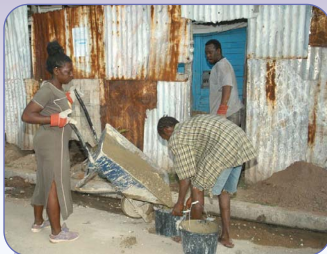
Construction activities underway
